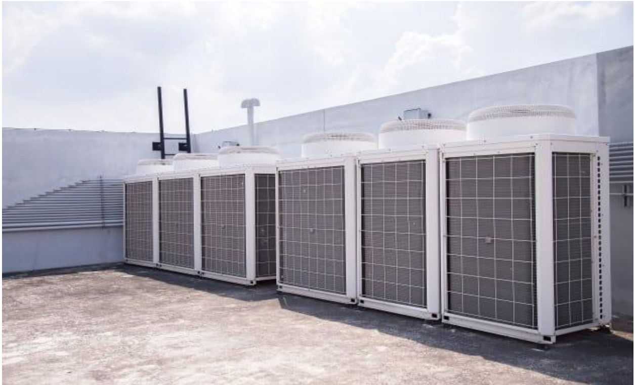
VRV Unit Installation
