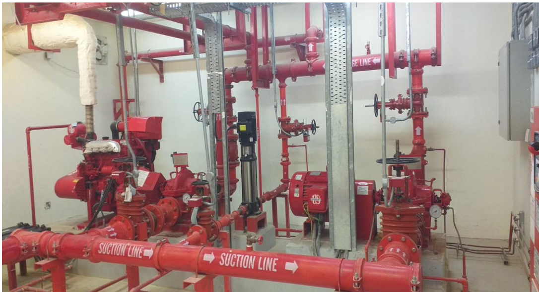
Fire Fighting Work
