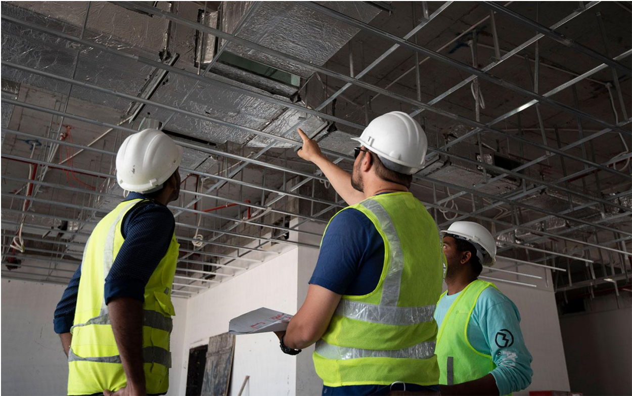
Duct & Ventilation Work
